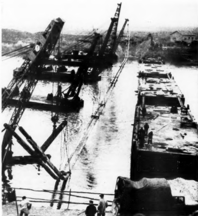
NEW LINE IN EUROPE. —One of the first important pipe lines to carry petroleum products in Europe is scheduled to go into service the latter part of this year. It is the 140-mile, 25-cm. (about 10-in.) line connecting the refinery area of the lower Seine with Paris. The line is designed to move about 31,000 bbl. daily of light products into 22 terminals between Colombes and Juvisy in the Paris area. The government, directly and through state-controlled interests, is the majority owner of the line; other shares are held by the refining companies involved. Black products will continue to be shipped by river barge. Shown here is the crossing of the Seine River between St. Denis Island and suburban Argenteuil by a double section of the line (Acme photo).
